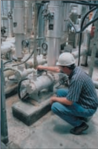
Typical installation of a Teikoku canned motor pump in a high temperature application.
